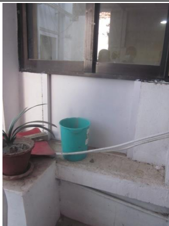
Figure 3: Misplaced bucket from ward
